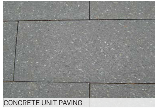
CONCRETE UNIT PAVING
